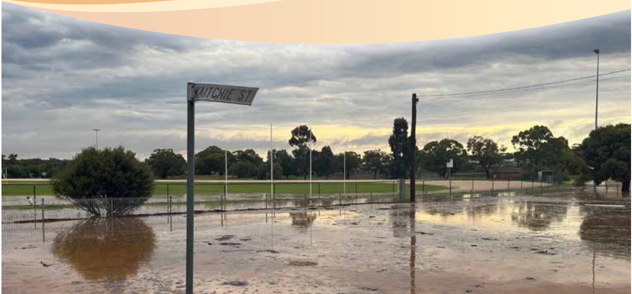
Flood damage in Waitchie Street, Wedderburn, 2023/24 flood event
