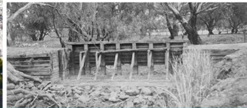
Kinypanial Creek weir constructed in the early 20th century
