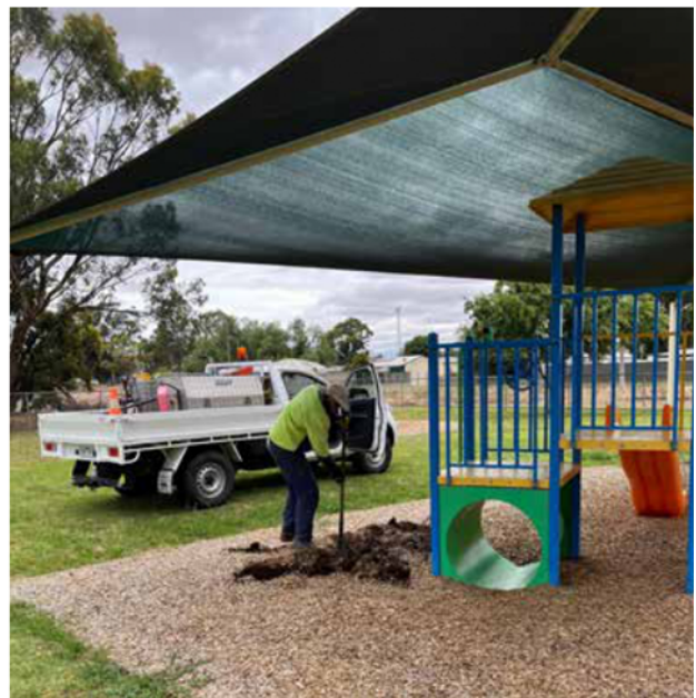
Maintenance work at Bridgewater playground.
