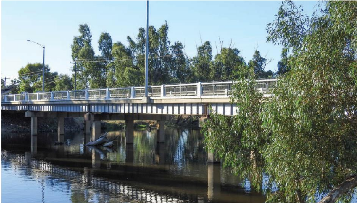
Bridge across the Loddon River, Bridgewater on Loddon
