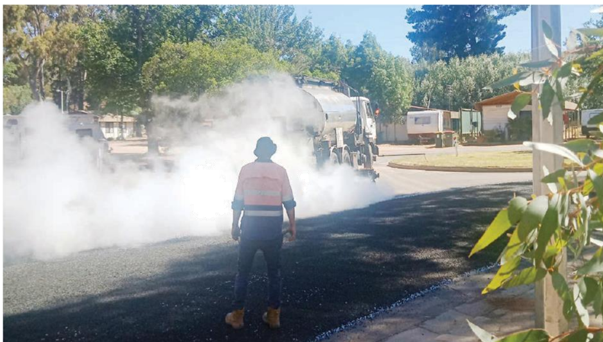
On-ground works underway at Wedderburn Pioneer Caravan Park.
