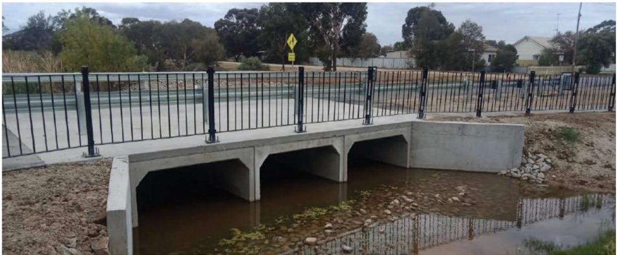
Culvert Replacement, Kelly Street Pyramid Hill.
