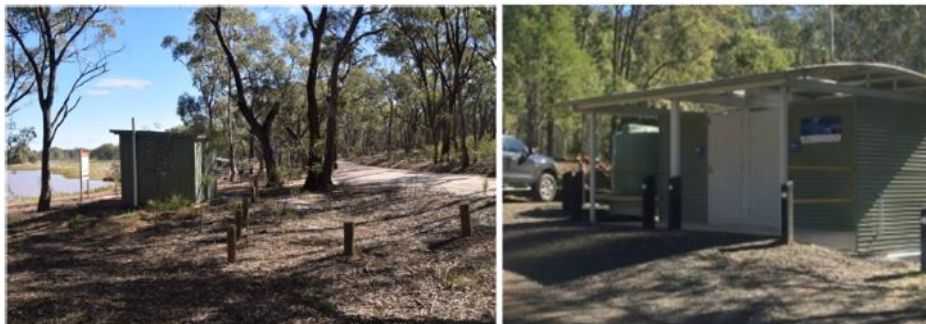
Figure 7.2 Existing drop-toilet at Skinners Flat Reservoir. Right: Example of a Dry Vault Toilet System.
