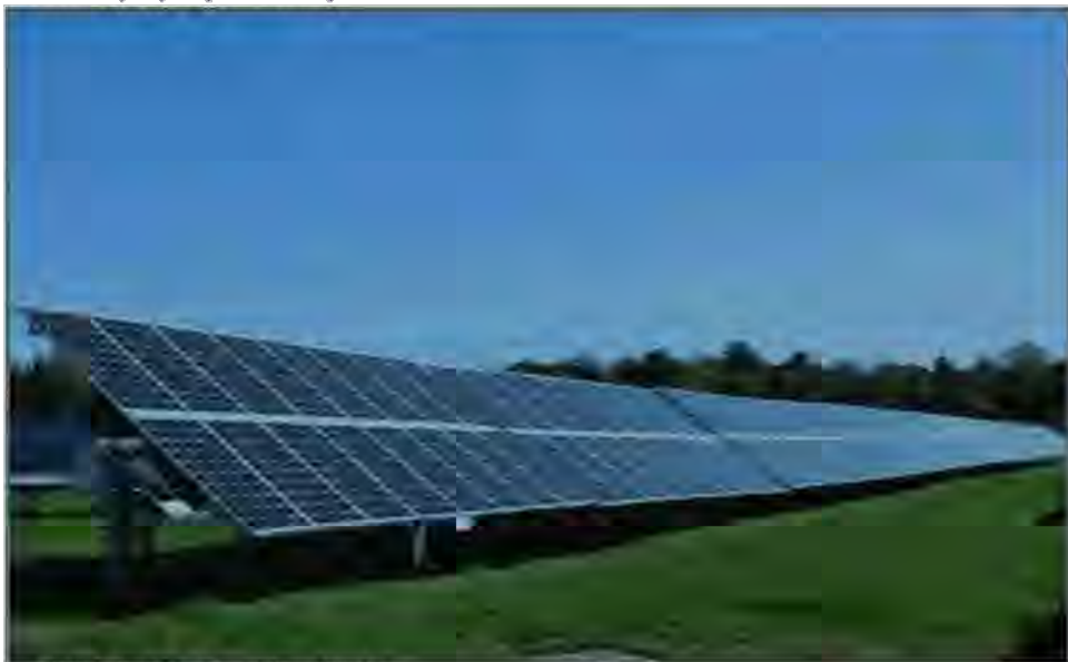
Example of Single Axis Tracking System
