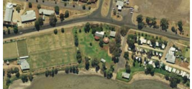
The Boort Eastern Entry Project begins.
