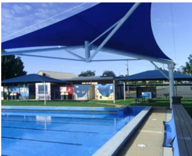
Loddon Shire Council's pools receive shade structures.
