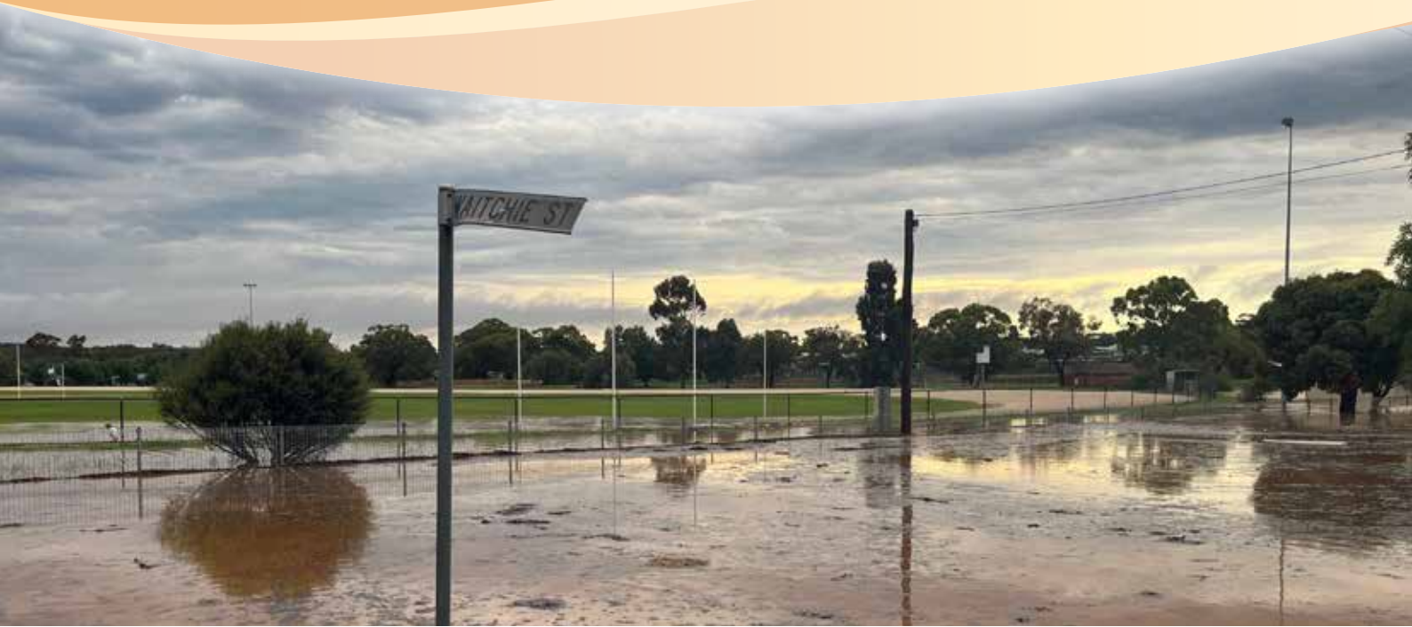
Flood damage in Waitchie Street, Wedderburn, 2023/24 flood event
