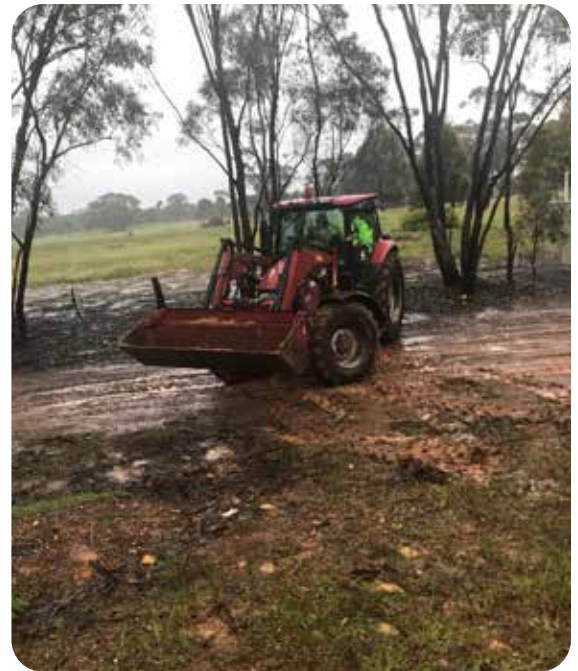
Flood works at Skinners October 2022.
