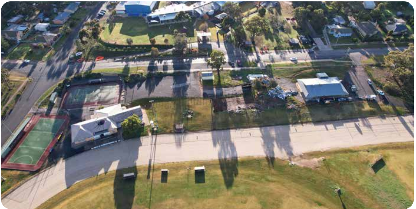
Demolition works begin at Donaldson Park.
