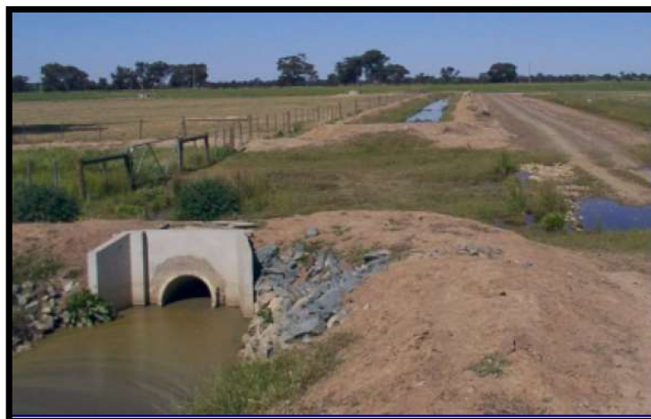
Figure 8 – Example of constructed siphon (Source: WFP Guidelines 2003)
