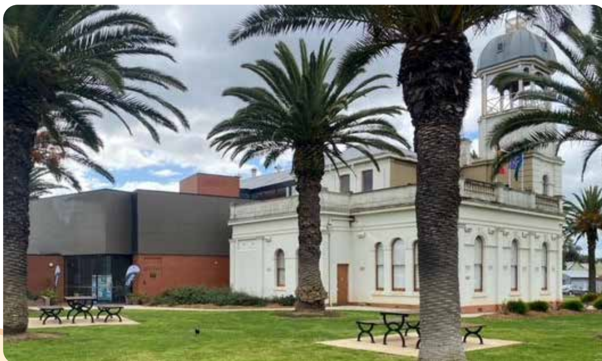
Inglewood Town Hall Hub.
