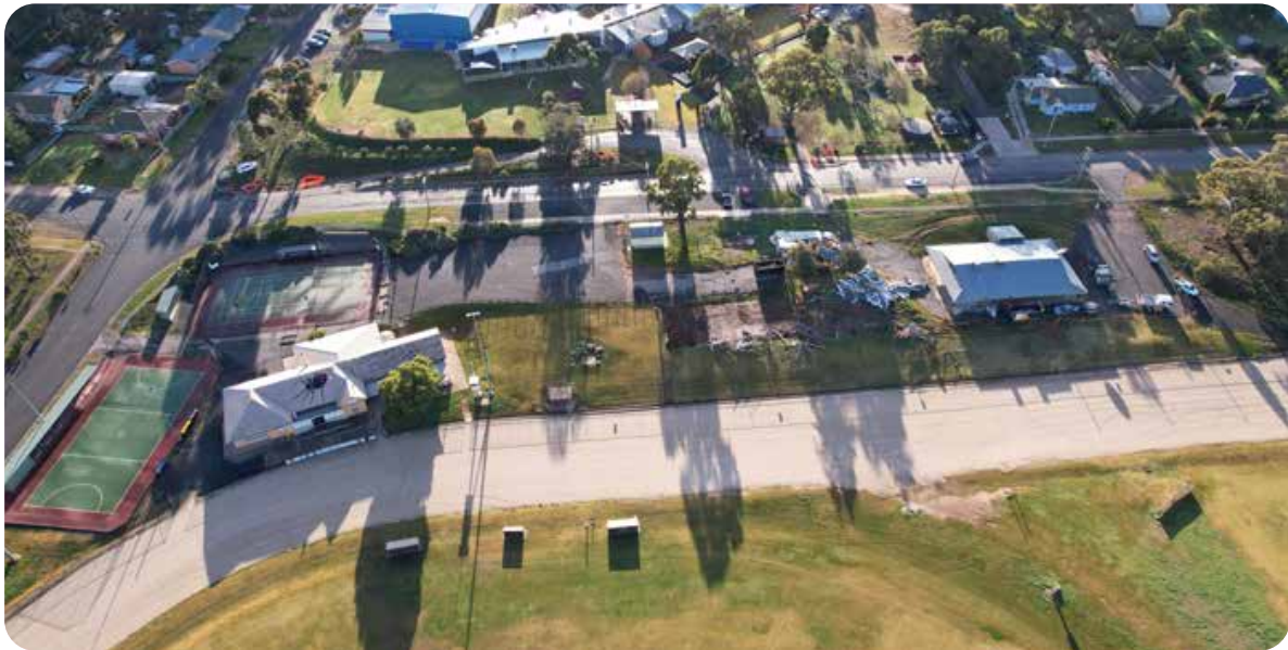
Demolition works begin at Donaldson Park.
