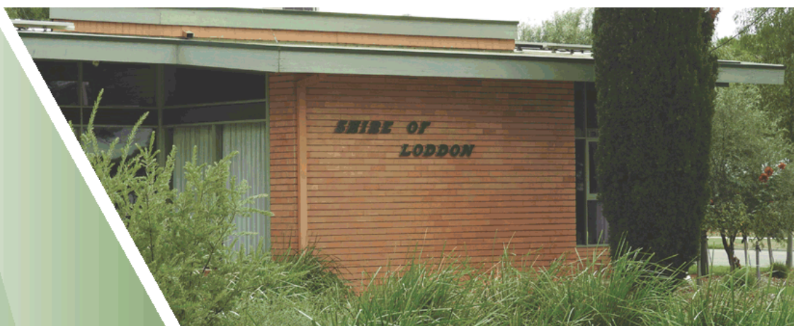
Council office at Serpentine.
