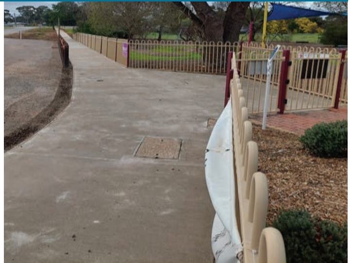
Footpath construction works in Southey Street, Inglewood have been completed.
