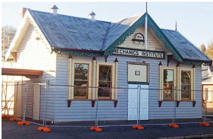
Restoration works at the Korong Vale Hall are nearing completion.
