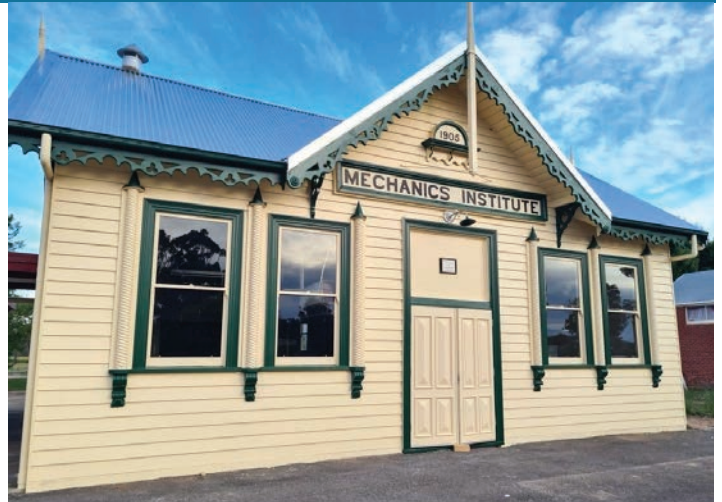
Restoration works at the Korong Vale Hall have been completed.
