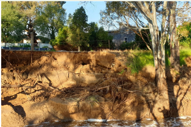
Bank erosion, Bullock Creek at Yarraberrb, October 2022 (image courtesy of Chris Heatherton)
