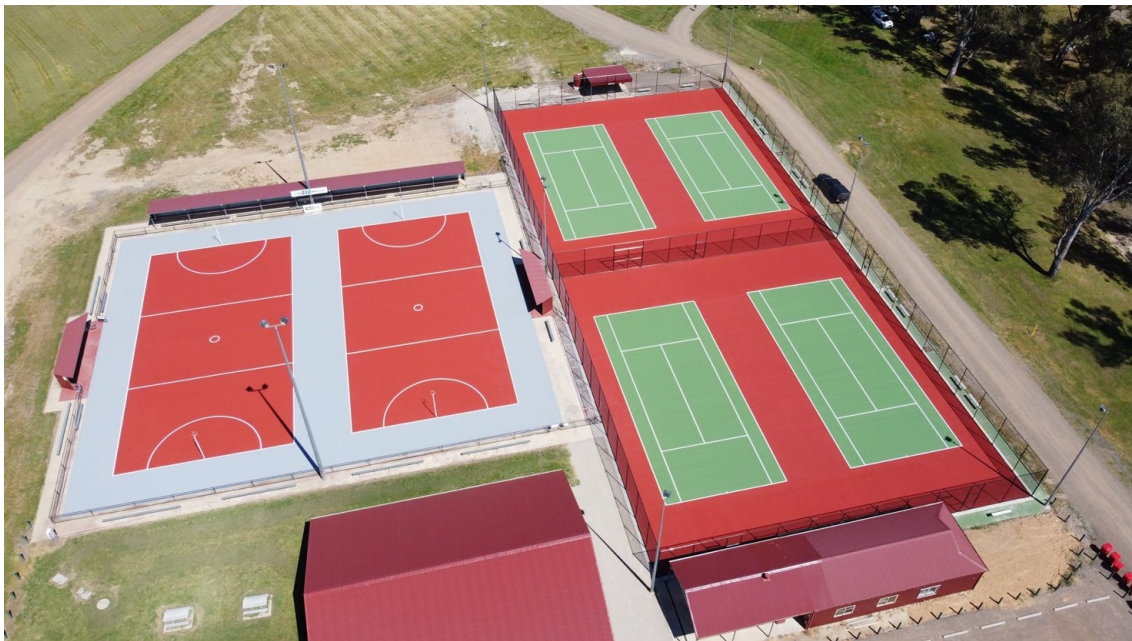
Figure 54: Newbridge Recreation Reserve
